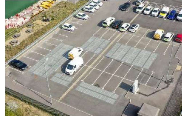
Dalles photovoltaïques Wattway by Colas
